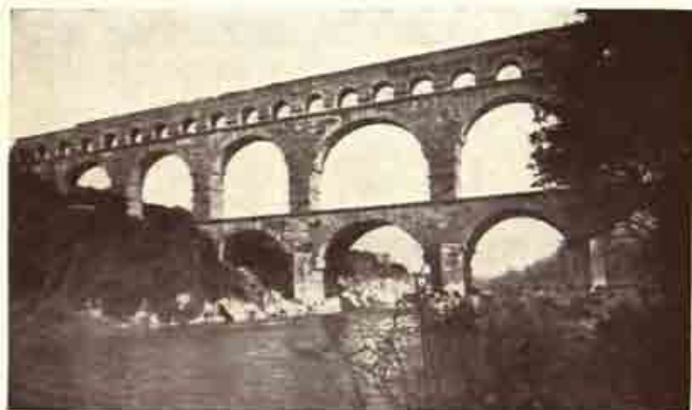
Pont du Gard, the Roman aqueduct which conveyed water to Nîmes from springs 25 miles distant. The water channel is above the highest series of arches (page 81)
