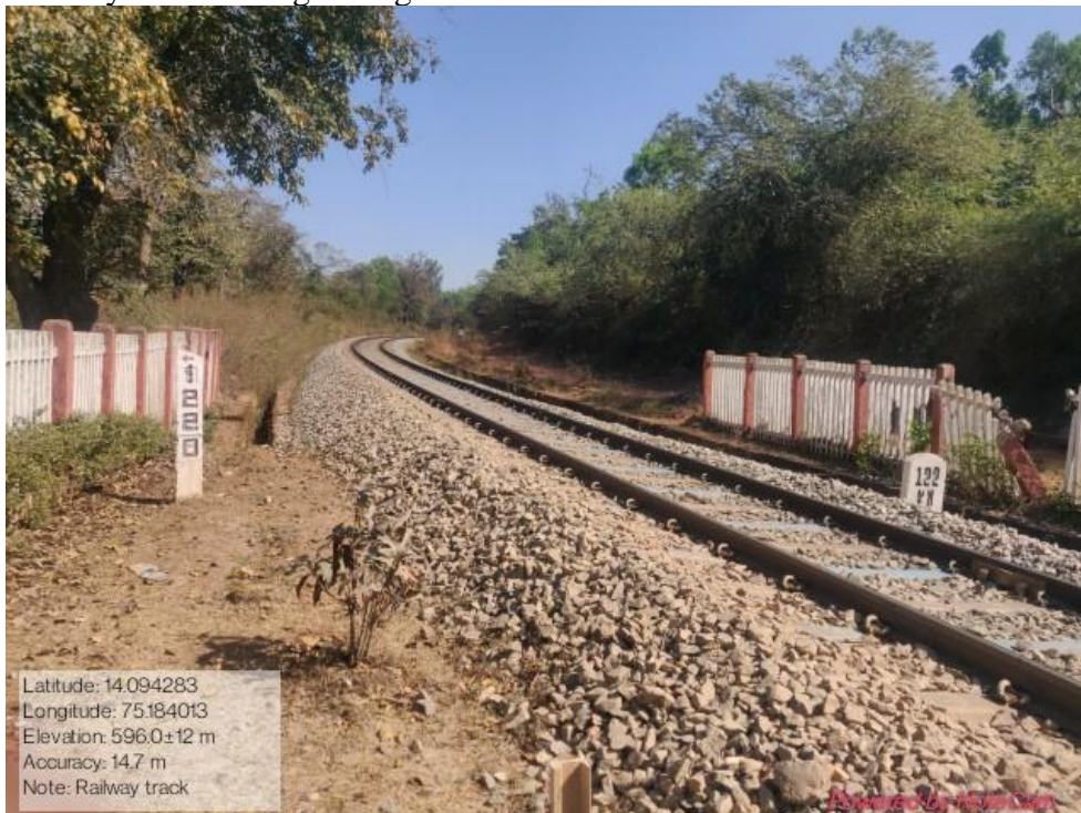
Railway track cutting through forest
