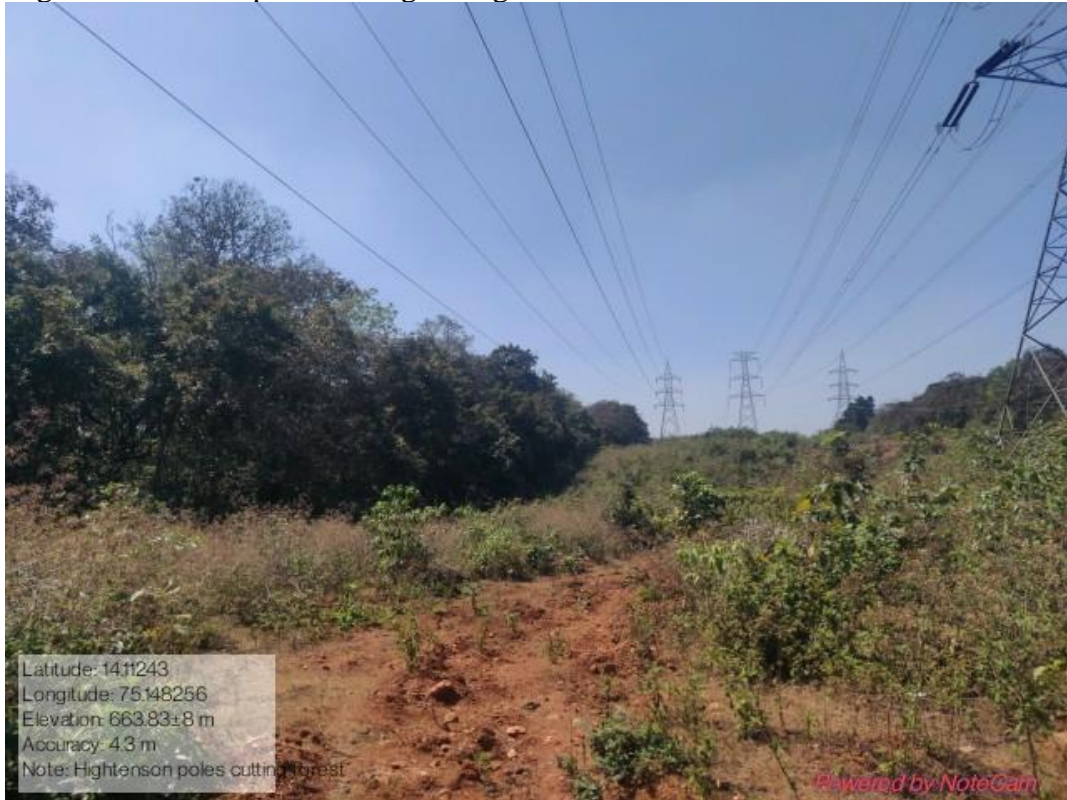
High Tension wire poles cutting through forest
