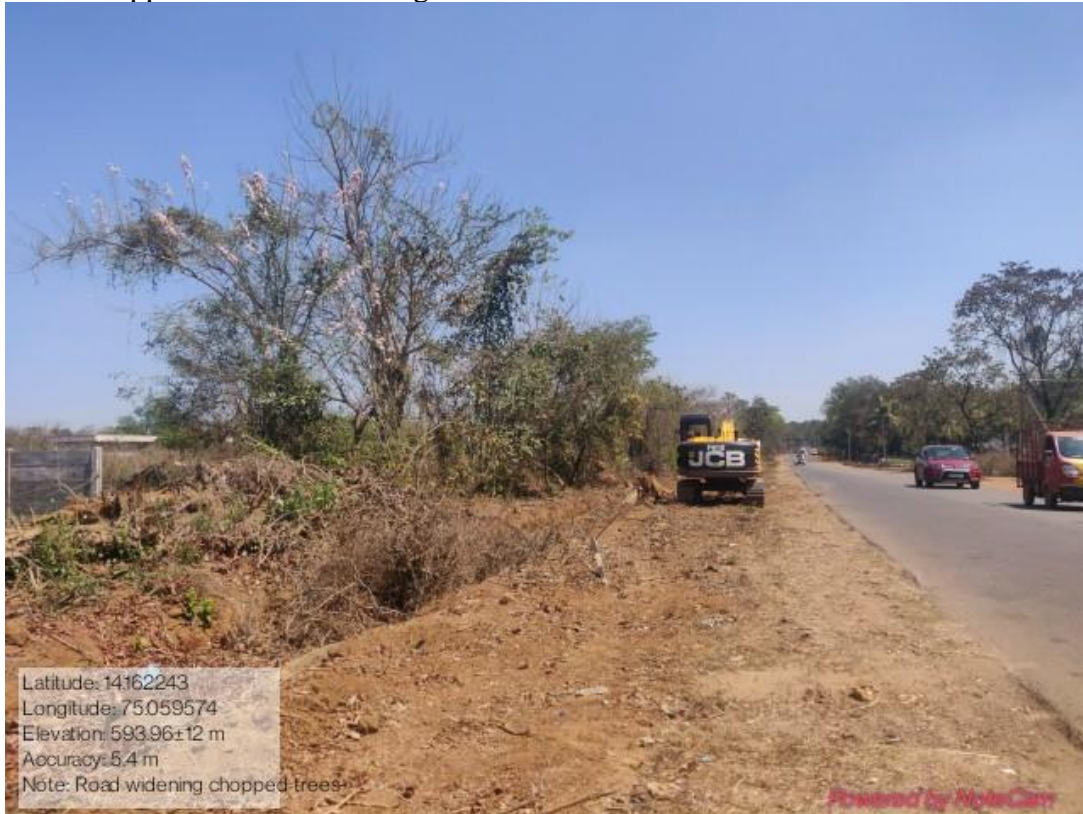
Trees chopped for road widening
