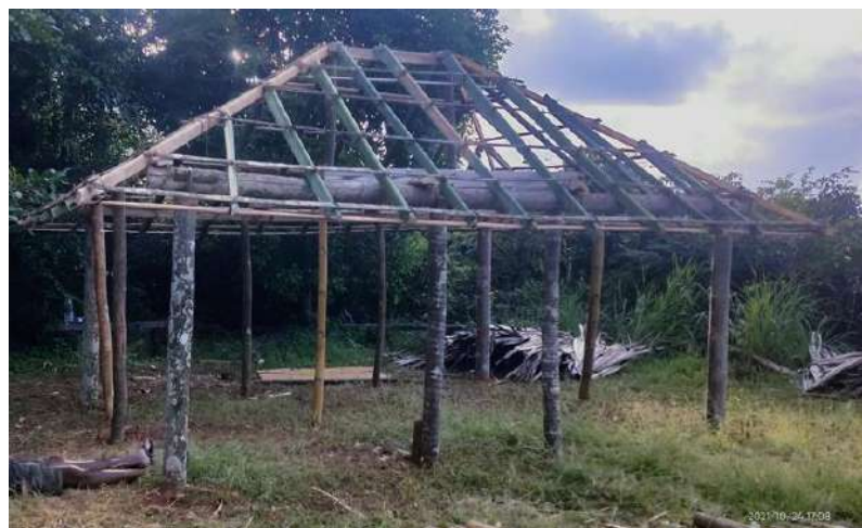
Photograph 3.3: Traditional House of the Mavilan Community Under Construction
